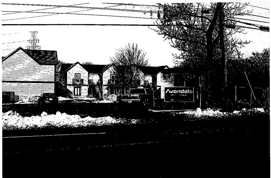
New construction finally gets underway at Adsum Court (December, 2005).
